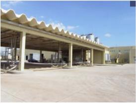
sealed from the inside as well as the outside. The "in situ" concrete was used in the super structure of the Spray / Mix building, the structure of the surveillance, cistern, basins and water tank.
